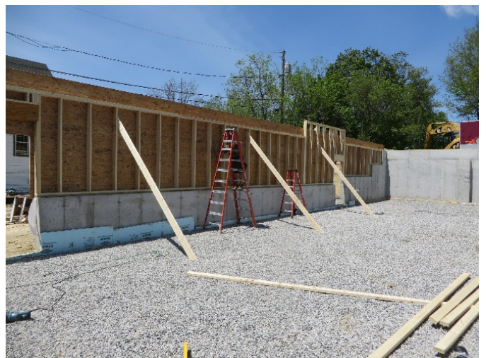
Framing the First Floor, 5-22-2019
