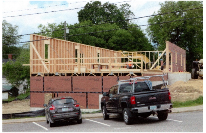
Framing Walls for Second Floor, 6-14-2019
