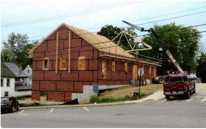
Installing the Roof Trusses, 6-19-2019
