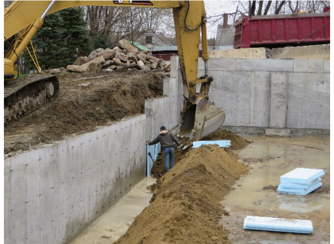
Insulating Interior of Foundation, 4-27-2019
