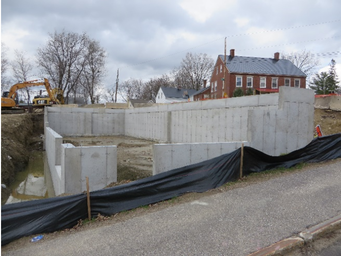
Foundation Walls Poured, 4-19-2019
