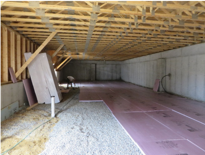
Installing the Floor Insulation, 7-12-2019
