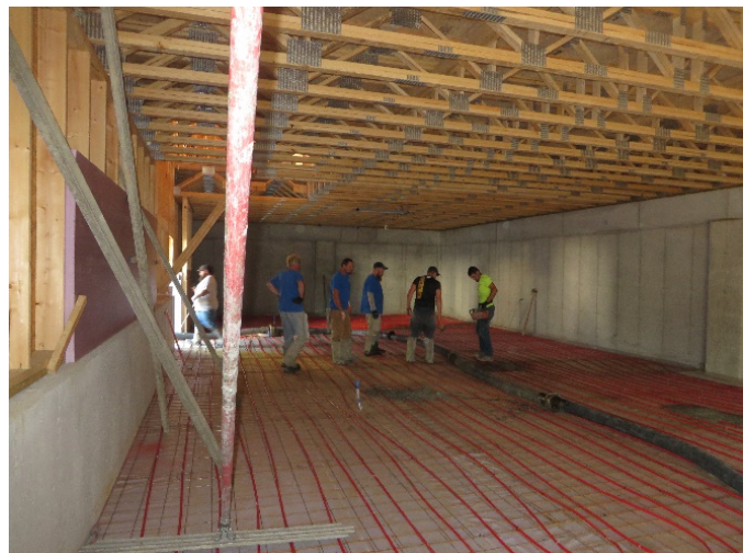
Installing the Radiant Heat Piping, 8-20-2019
