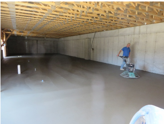
Finishing the Concrete on the First Floor, 8-26-2019
