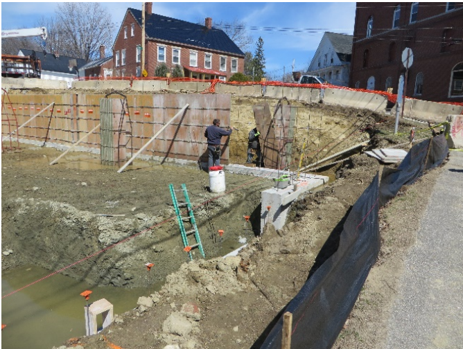
Installing the Forms for the Foundation, 4-11-2019
