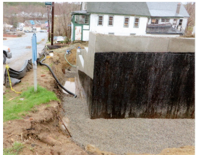
Stone Covering Perimeter Drain, 4-19-2019
