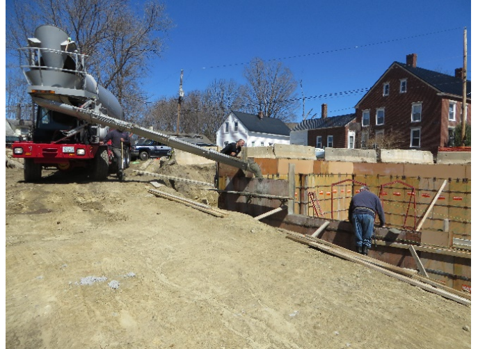
Pouring Foundation Walls, 4-17-2019
