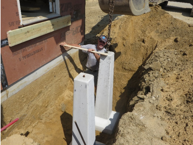
Installing the Porch Supports, 7-27-2019
